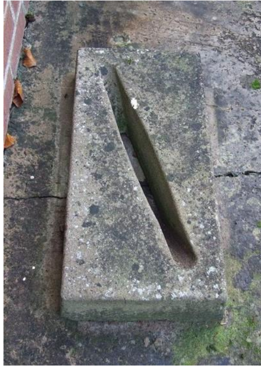
Concrete Cycle Support
