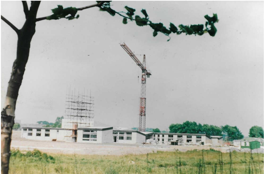
Eccles College Under Construction in 1971
