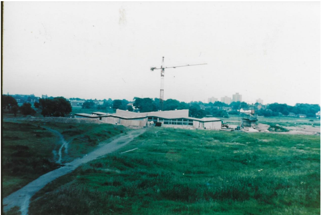
Eccles College Under Construction in 1971
